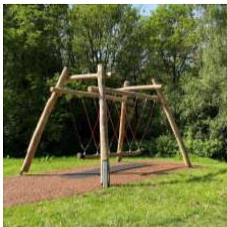
**Above:** Broadstone Recreation ground, high quality rope and rope fixings, a wear pad installed under the new rope swing will ensure long-term durability of the surfacing in a high friction zone.
